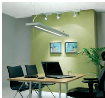
Fluorescent lighting louver in internal office
